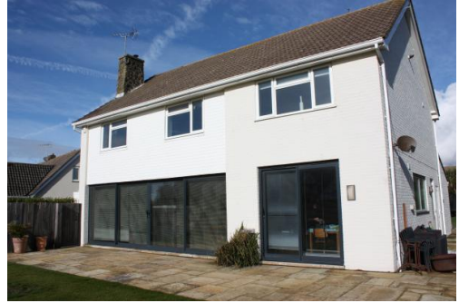
Image 4. The front of the house viewed from the garden.
