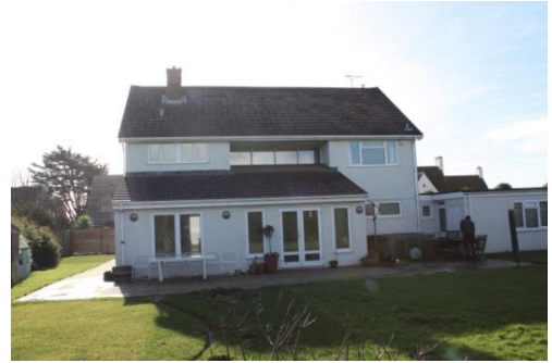
Image 3. The North elevation of the house.
