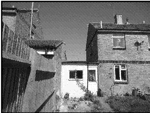
Rear Elevation of 86 & 84 Roundstone Drive.
