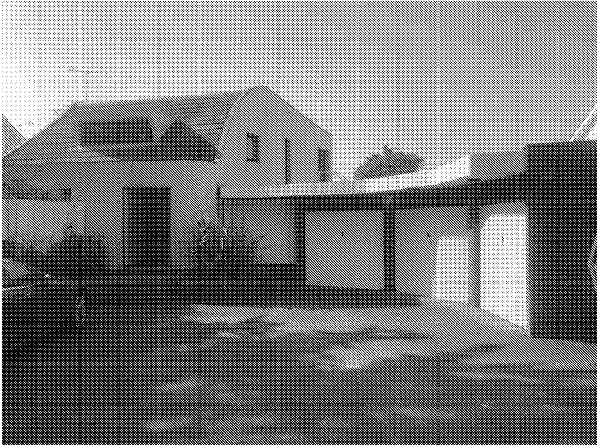
Views of Vista Point from Tamarisk Way showing 3 garage doors
