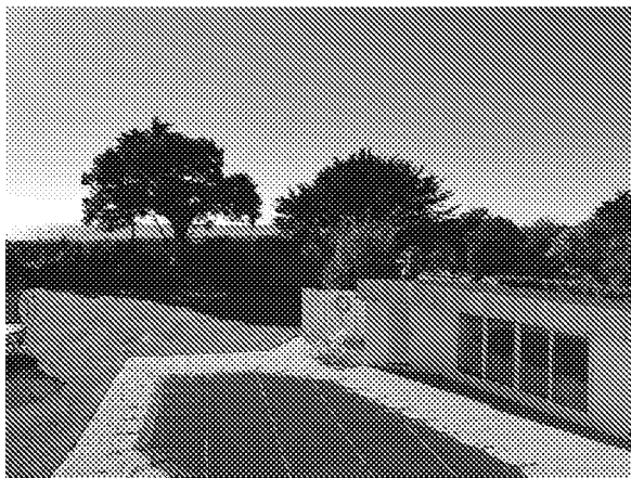
Existing view of pool and adjacent pool building
