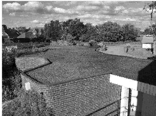
View over the roof of the garages
