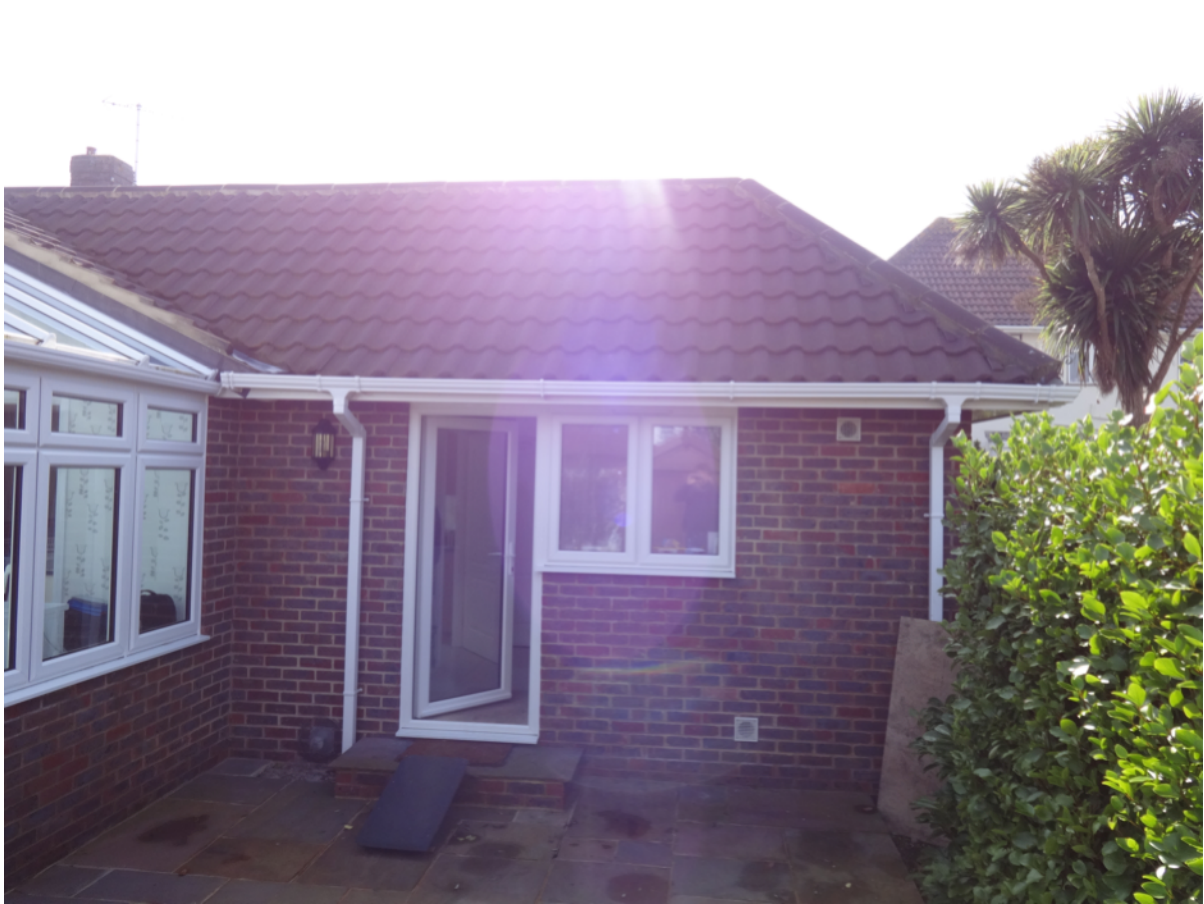
UTILITY BEHIND EXISTING GARAGE
