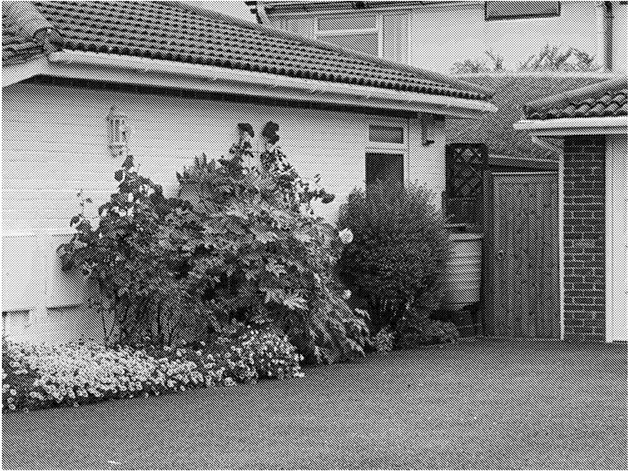
Photo 3 - South Elevation of Dean House over Ash Hollow Garage - Small window in South Elevation annotated on Block Plan
