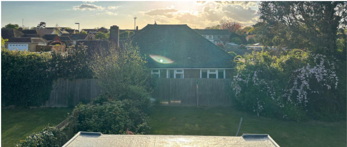
Image taken from the South end of the rear roof
