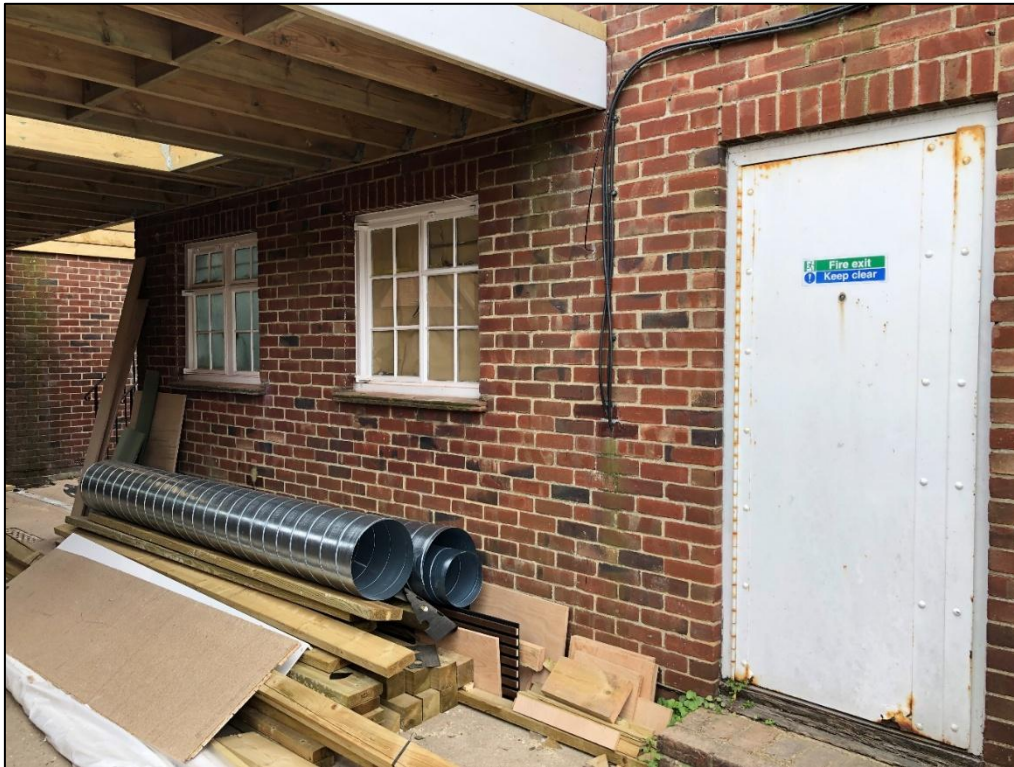
Figure 9. Installation location with Shelter.
