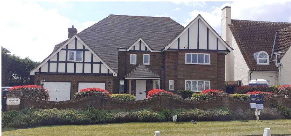
North Elevation (street view)
