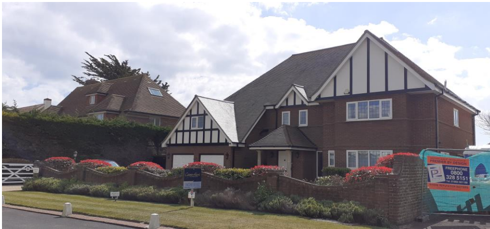
North West view
