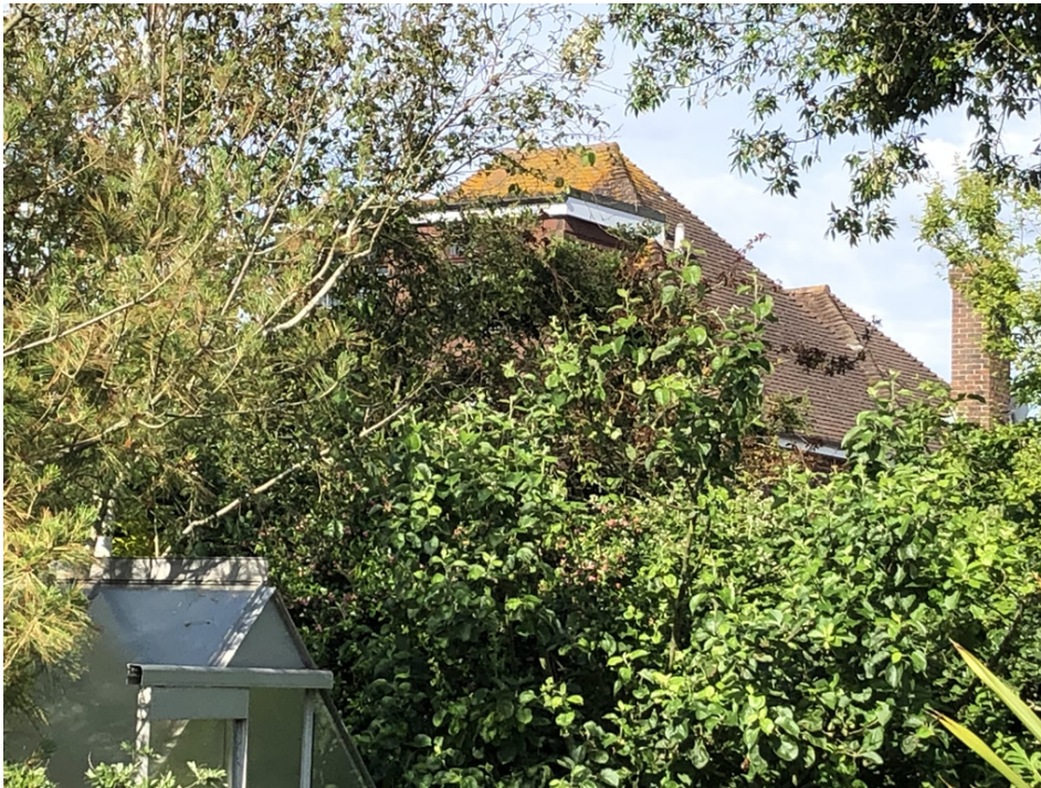
Large 3 storey property at 48 Sea Lane (directly behind no. 31 The Ridings) viewed from the garden of no. 33
