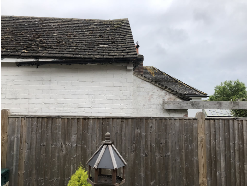
View from the back door of no 33 looking north (garage and outbuildings of no. 31 with main building behind and to the right)
