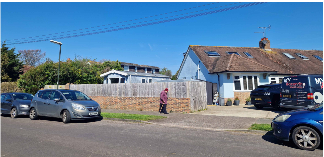
Photo 02 - Existing Street View
