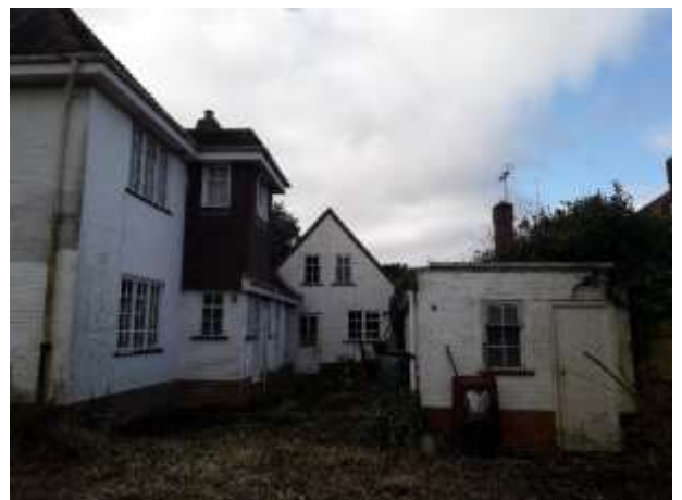
Side (north) / rear elevation
