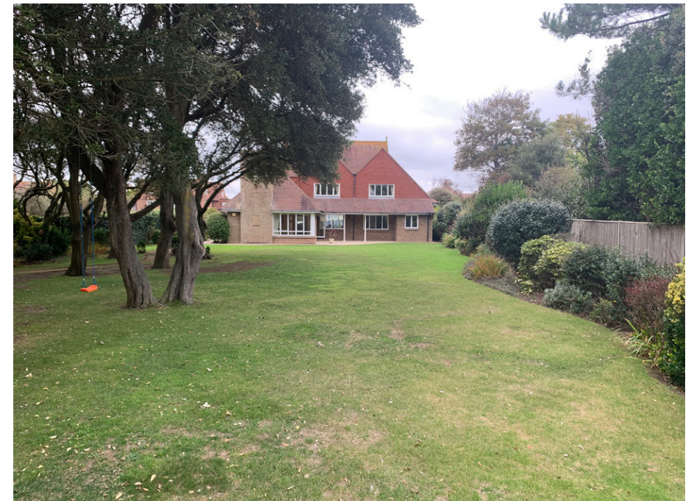
External view of existing building and rear garden – South elevation
