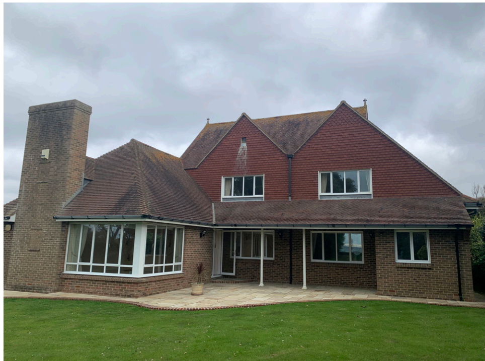
Exterior view of existing building – South Elevation
