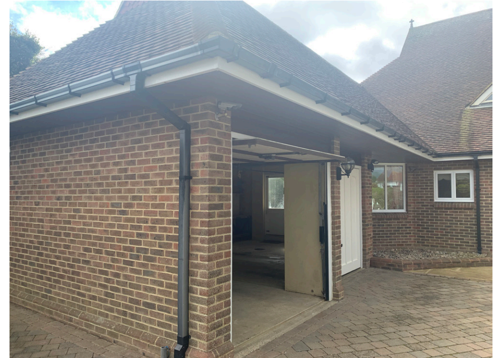
Exterior view of existing garage
