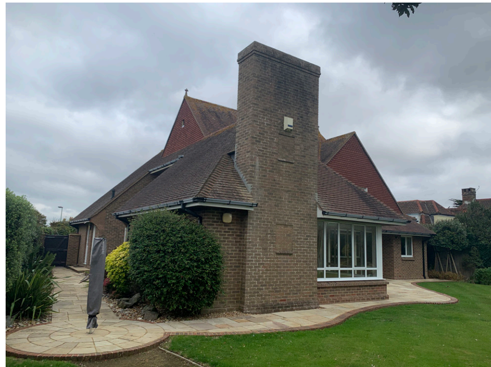
Exterior view of existing chimney
