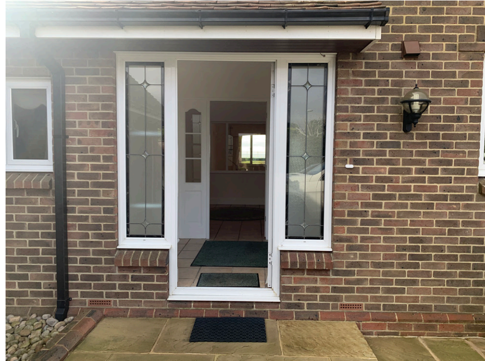
Exterior view of existing front entrance
