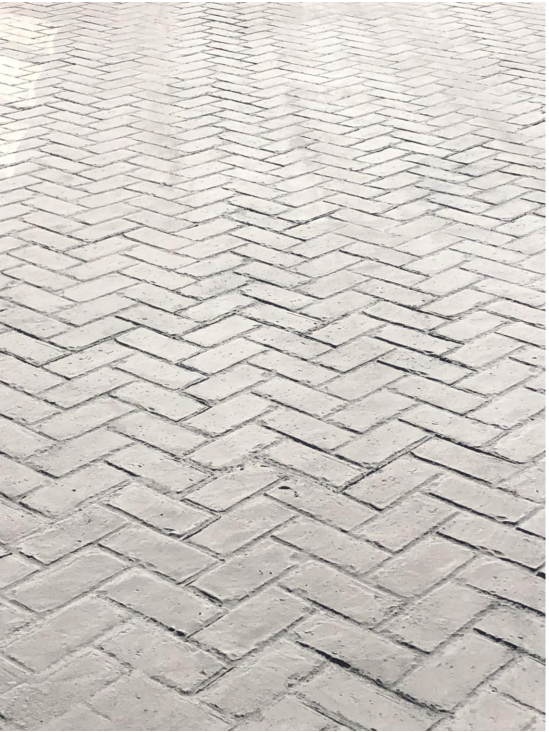
Outdoor paving (Herringbone)
