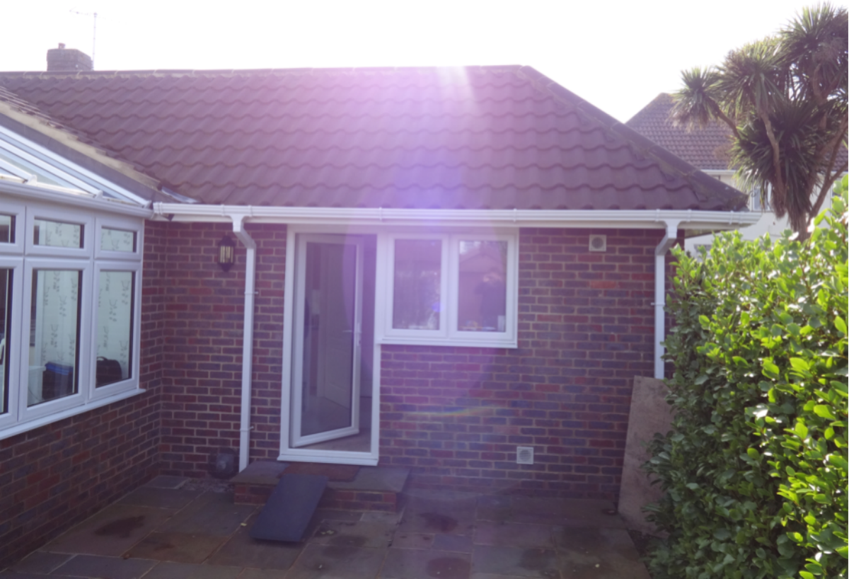
UTILITY BEHIND EXISTING GARAGE
