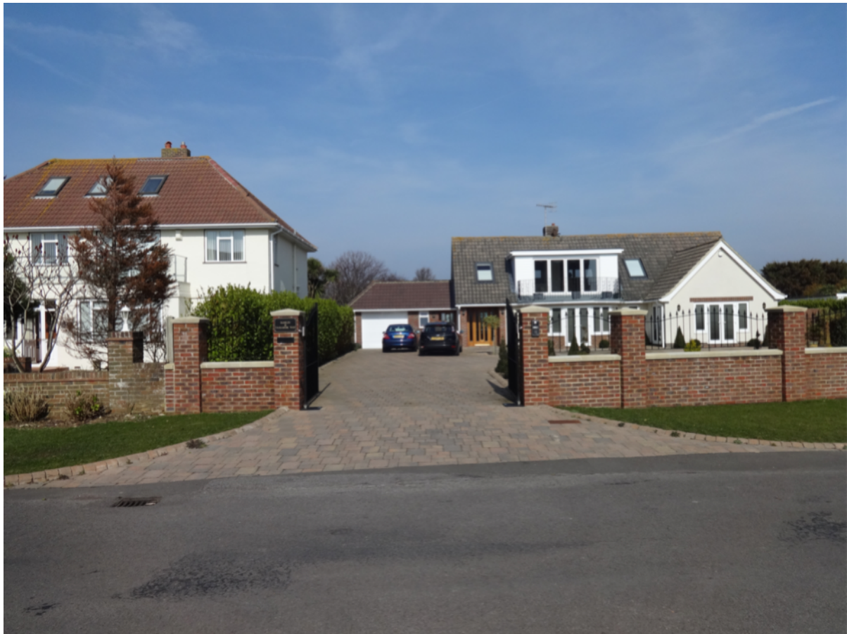
GENERAL VIEW FROM THE SOUTH
