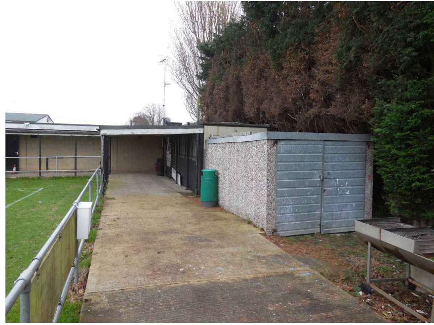
MARLEY GARAGE TO BE REMOVED
