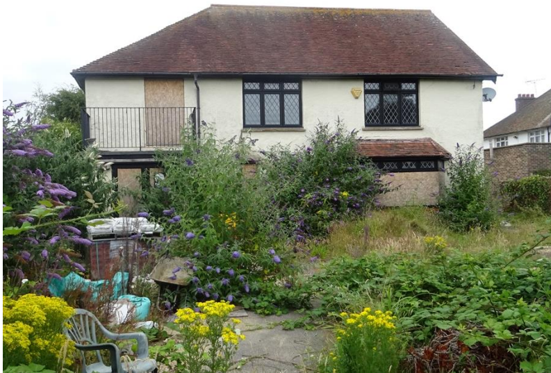
Figure 7: The Existing Building
