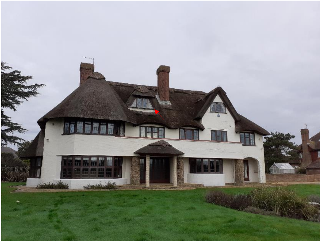
Photo 6: southern elevation of B1. Suitable bat roosting features indicated by red arrows.
