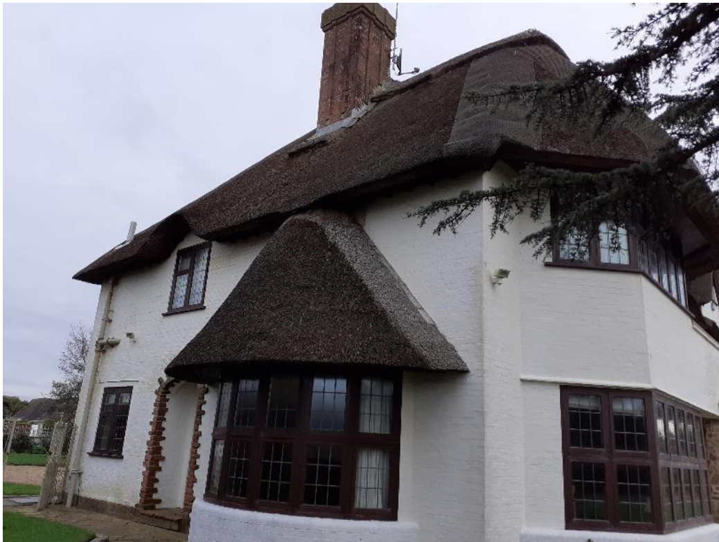
Photo 5: western elevation of B1, there are no suitable roosting features for bats on this elevation.
