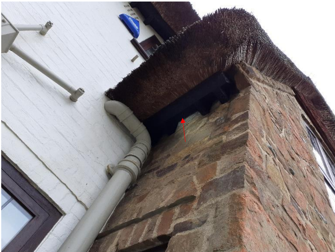
Photo 3: close up of the gap under the eaves of the northern gable end. The top eaves on this elevation appear to be tight fitting.
