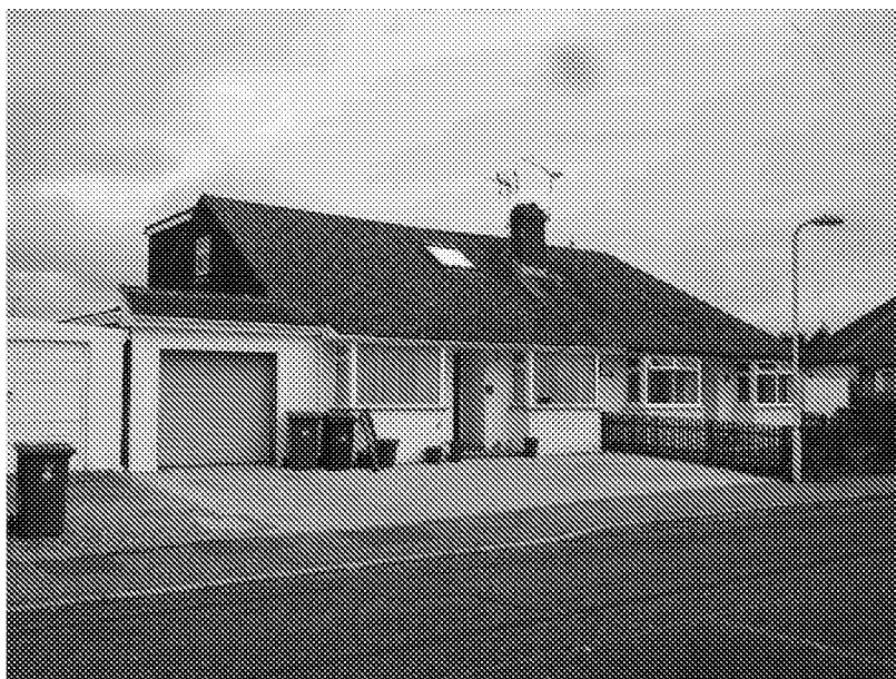
Photo 7. 59 Warren Crescent. Hip to gable loft conversion.
