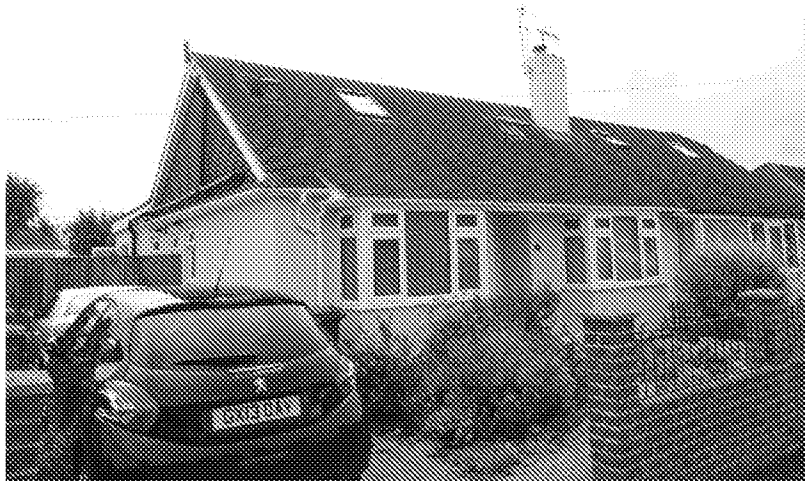
Photo 4. 22 Warren Crescent. Hip to gable loft conversion.
