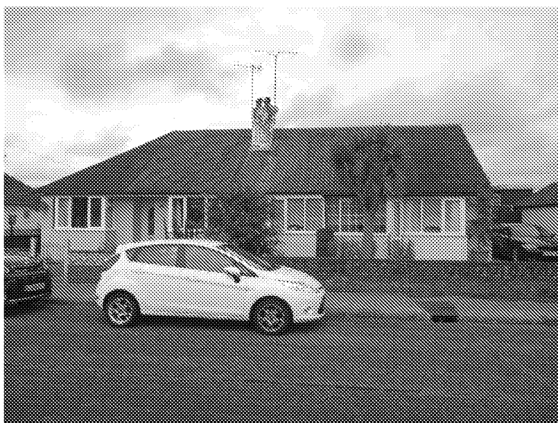
Photo 2. 13 Warren Crescent. Hip to gable loft conversion.
