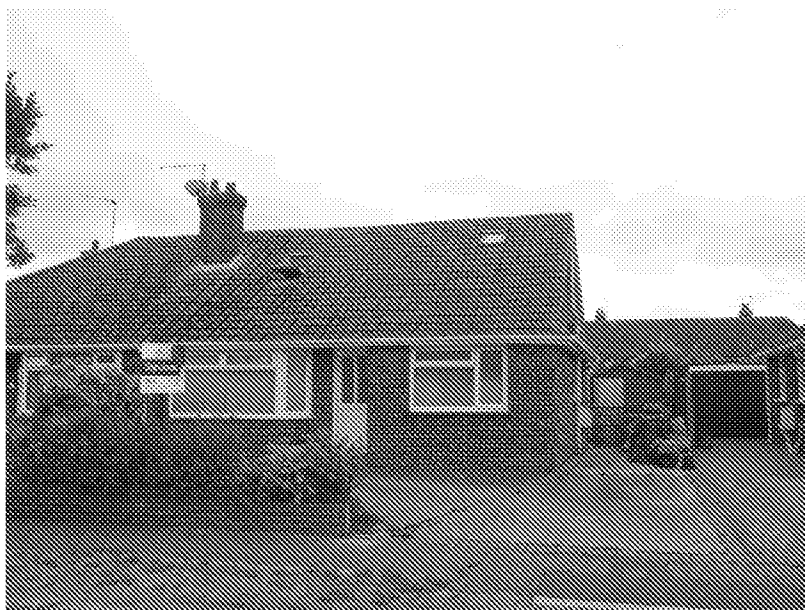
Photo 12. 33 Hillview Crescent.- (Only 2 doors down). Hip to gable loft conversion.
