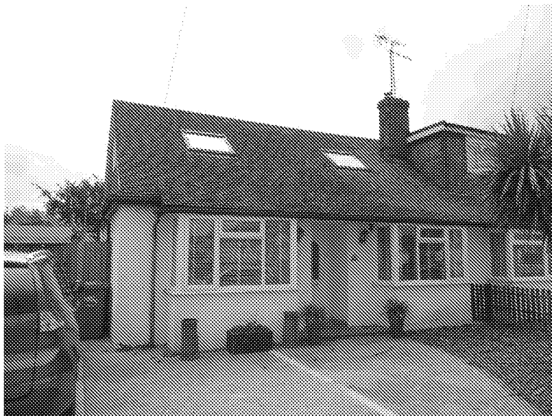
Photo 5. 30 Warren Crescent. Hip to gable loft conversion.
