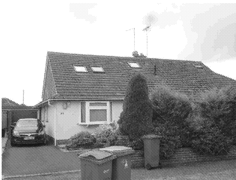
Photo 14. 44 Hillview Crescent. Hip to gable loft conversion.
