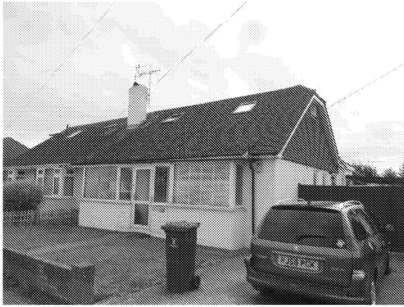
Photo 3. 20 Warren Crescent. Hip to gable loft conversion, with small barn end / half hip.
