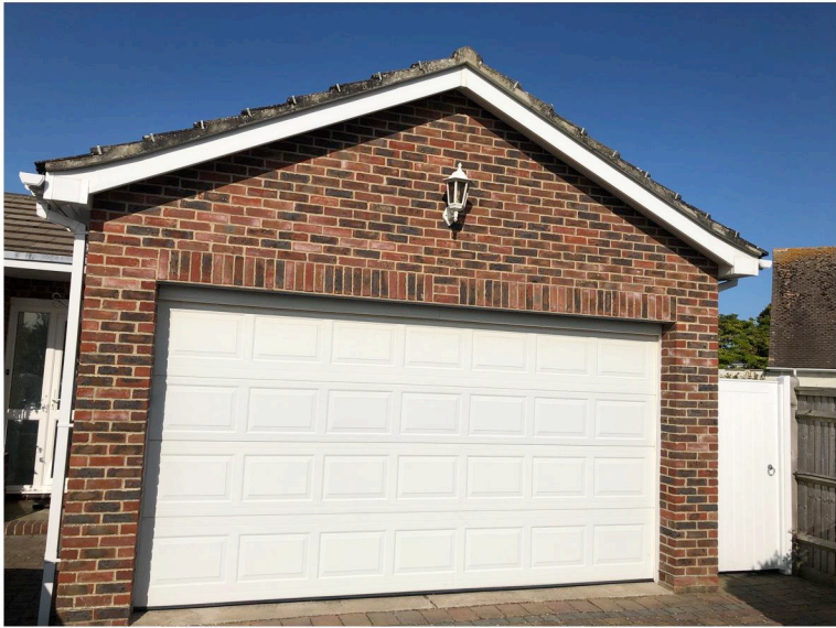
View of south east elevation [Garage to be extended]
