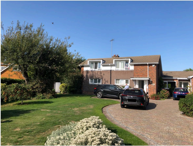
View of south east elevation
