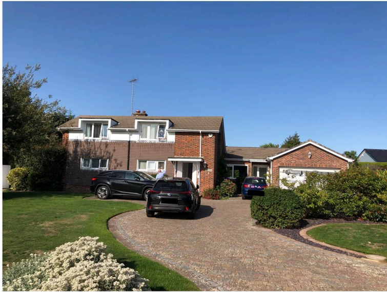
View of south east elevation [New Porch to Front]
