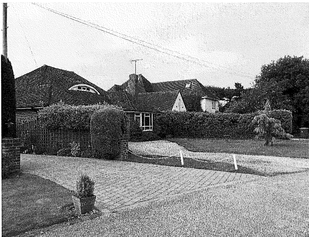
B. 43 and 45 Sea Lane, looking south. Council is concerned that the increased bulk on the northern side of 45 Sea Lane will be overbearing to 43 Sea Lane.
