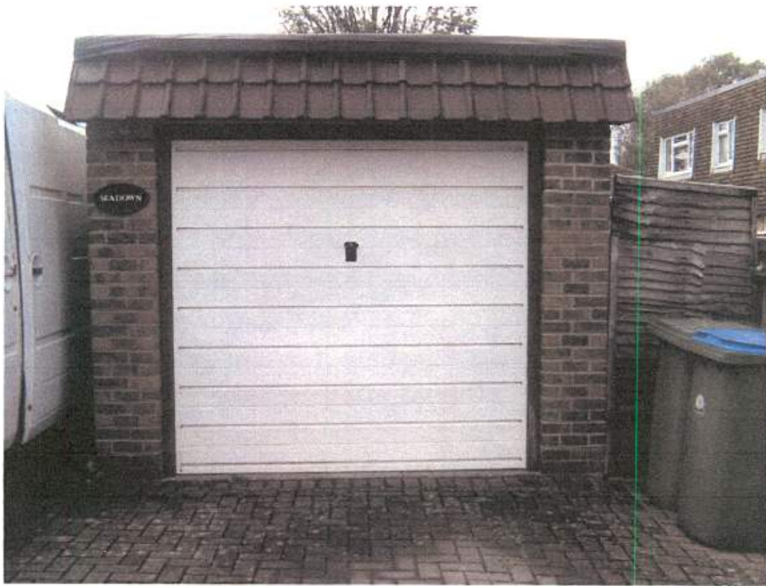
EXISTING GARAGE (EAST ELEVATION)
