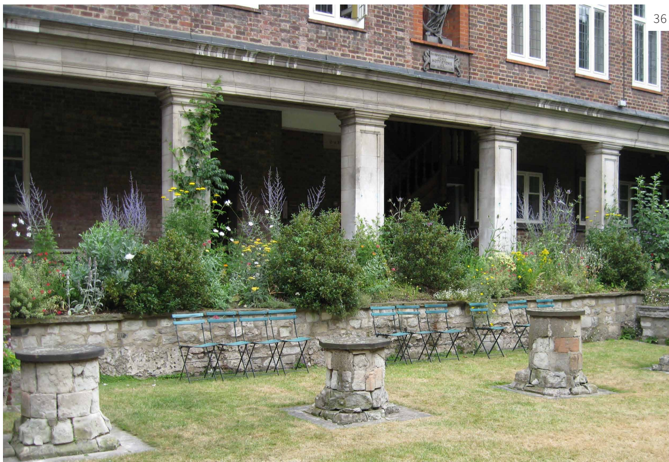
Figure 36 Trials of various consolidants (including nanolime) have been carried out on the remains of Reigate stone columns at Westminster Cathedral. These are part of the long-term monitoring of the effect of nanolime.
