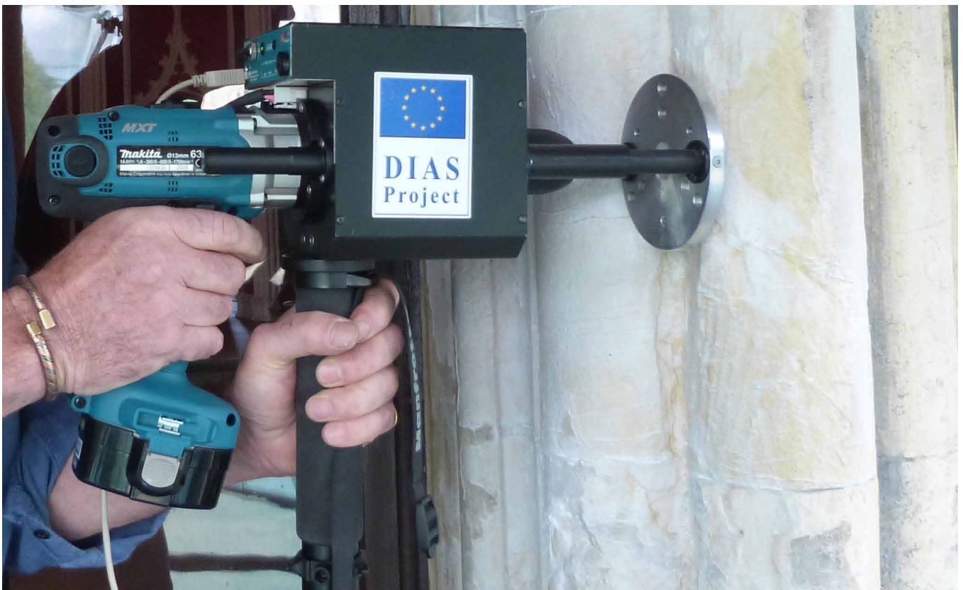
Figure 32 Using the Drilling Resistance Measurement System (DRMS).
