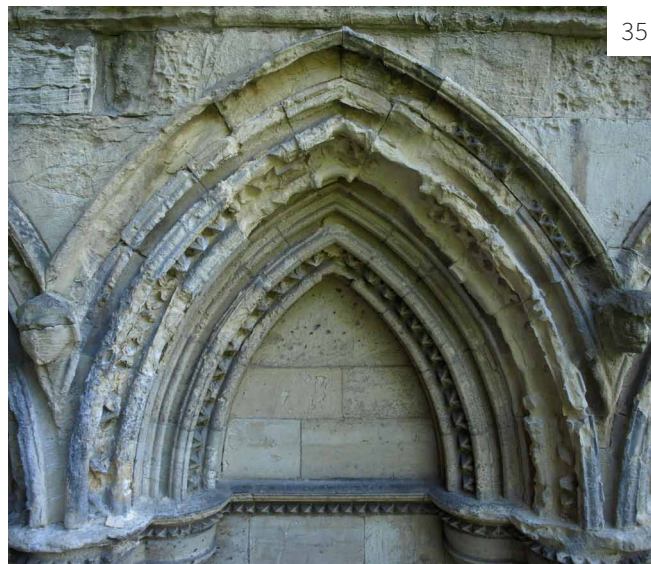
Figure 35 York Minster. This area was chosen to carry out trial repairs of the magnesian limestone. The results were sufficiently good to allow conservators to adopt nanolime as a pre-treatment (prior to mortar repair and shelter coat) for decayed areas of stone on the East Front of the Minster.
