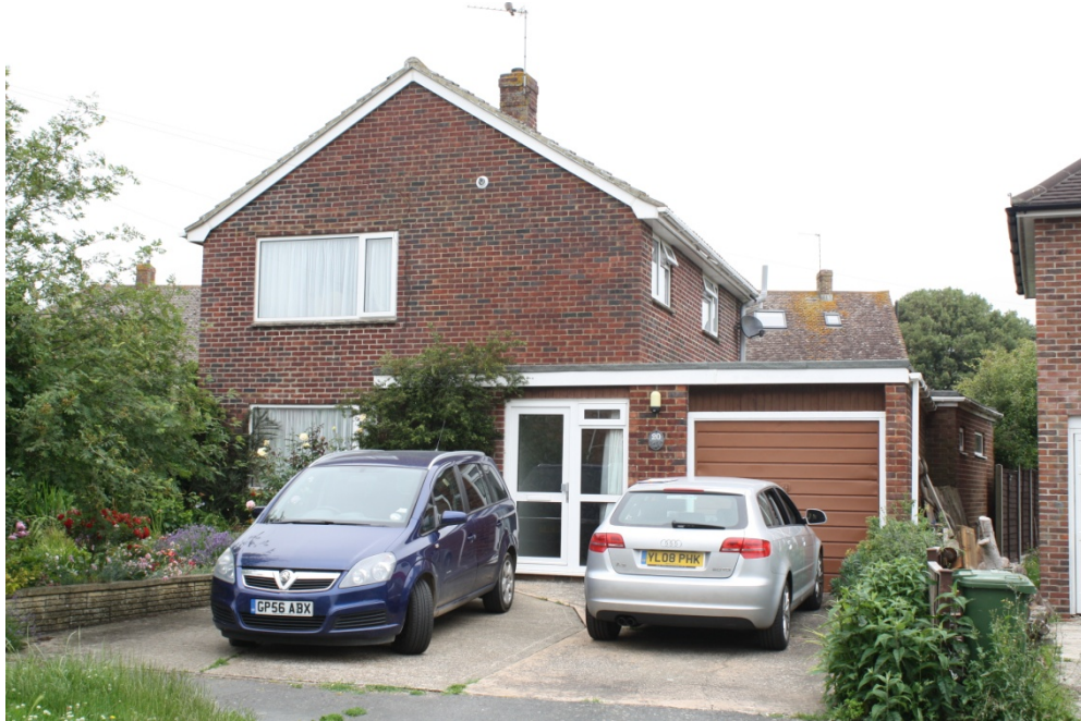
FRONT ELEVATION OF EXISTING BUILDING
