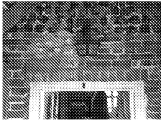
Figure 5: Shows existing front door and lintel to be raised. Brickwork to be salvaged and re-used.
