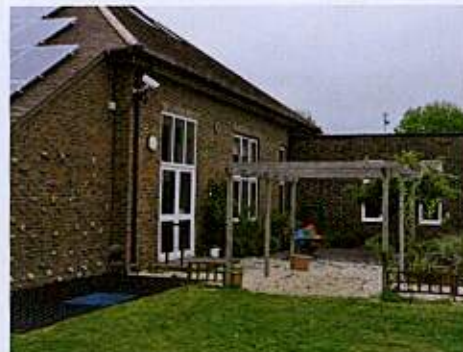
Brickwork on existing school hall
