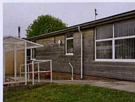
Timber cladding on brick plinth to existing school entrance and offices.
