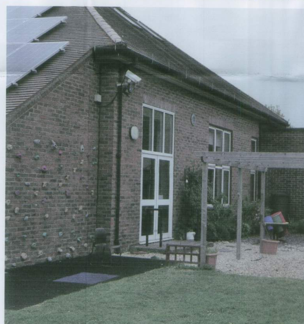
Chailey Rustic Stock Brick from the Existing School Hall
