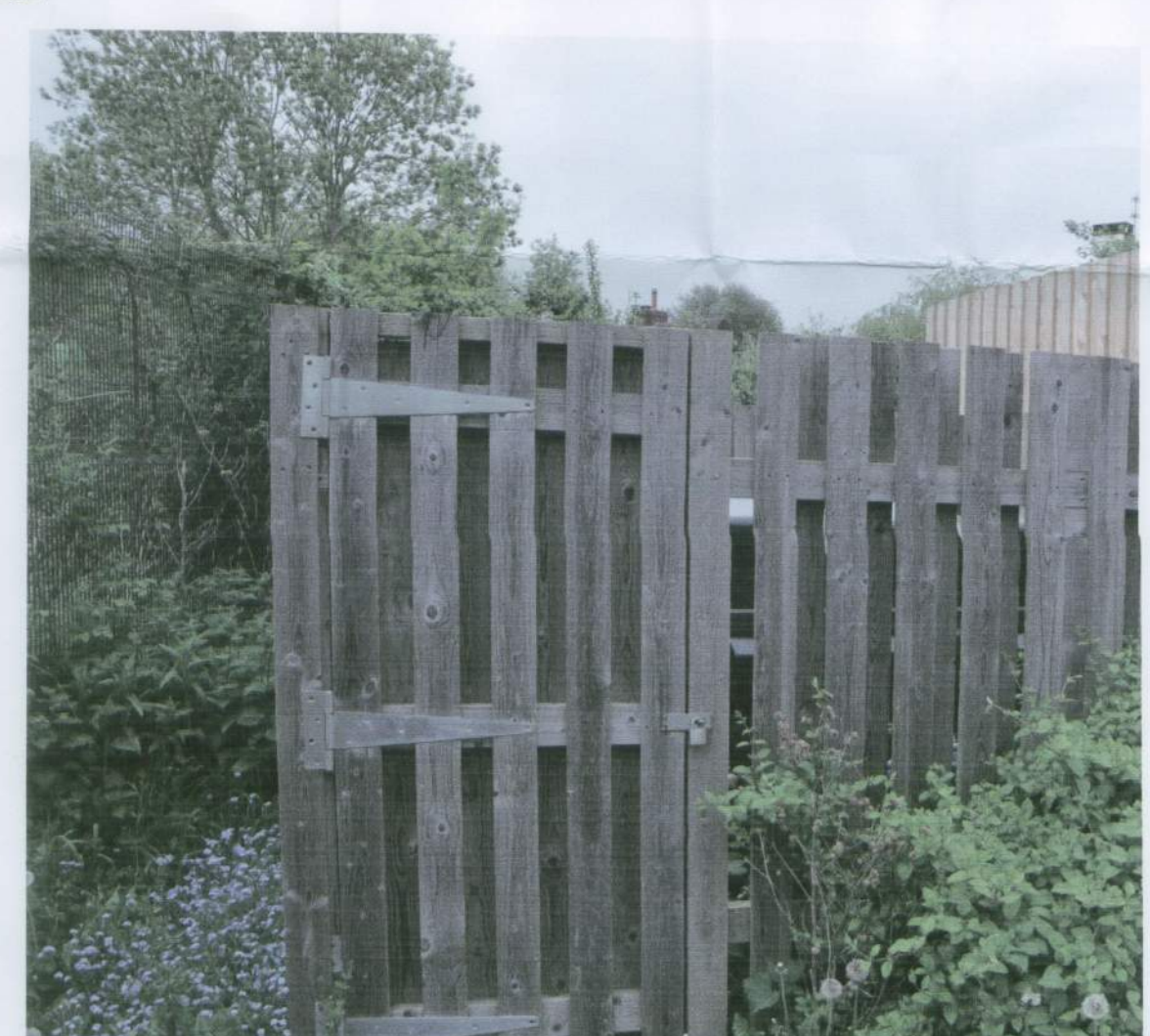
Green Weldmesh Fencing and Hit & Miss Fencing as seen at the Existing School
