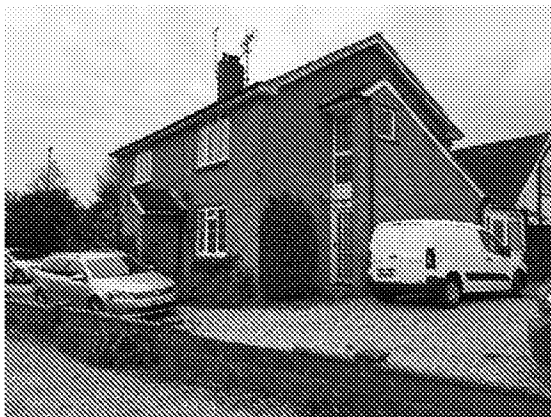
View of the existing northeast elevation of the house.
