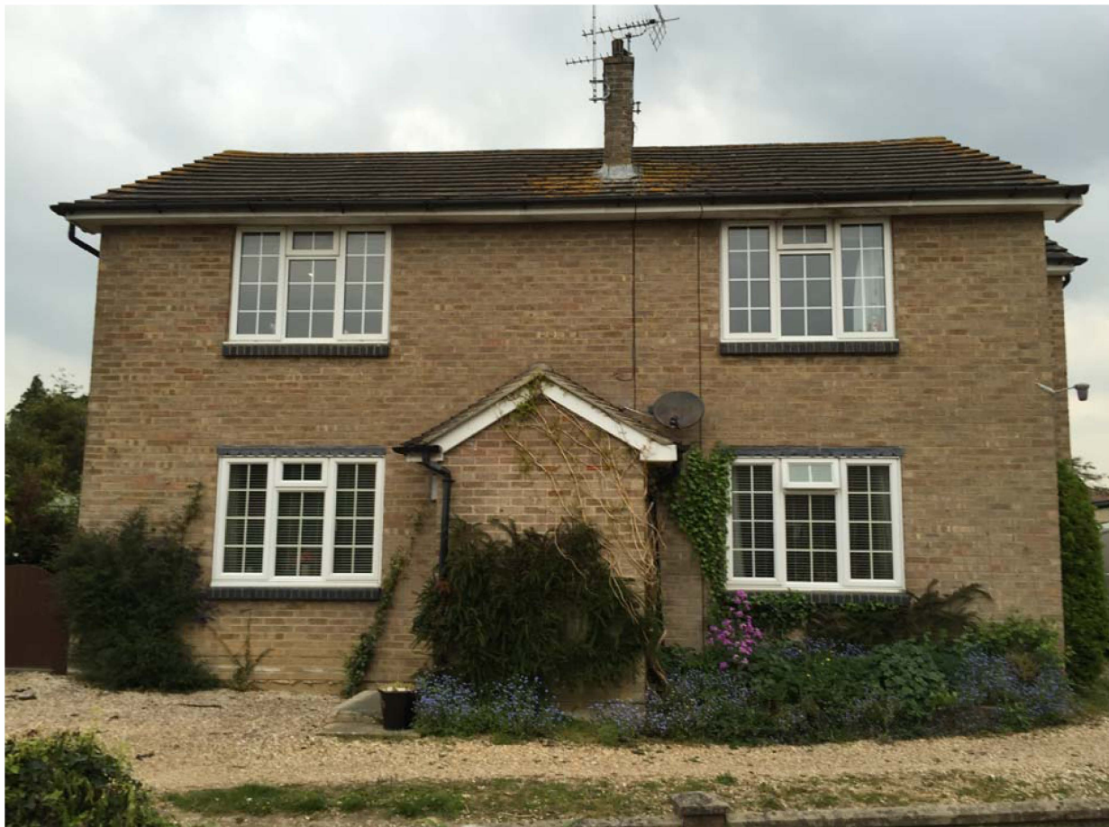
View of House from the South - main elevation
