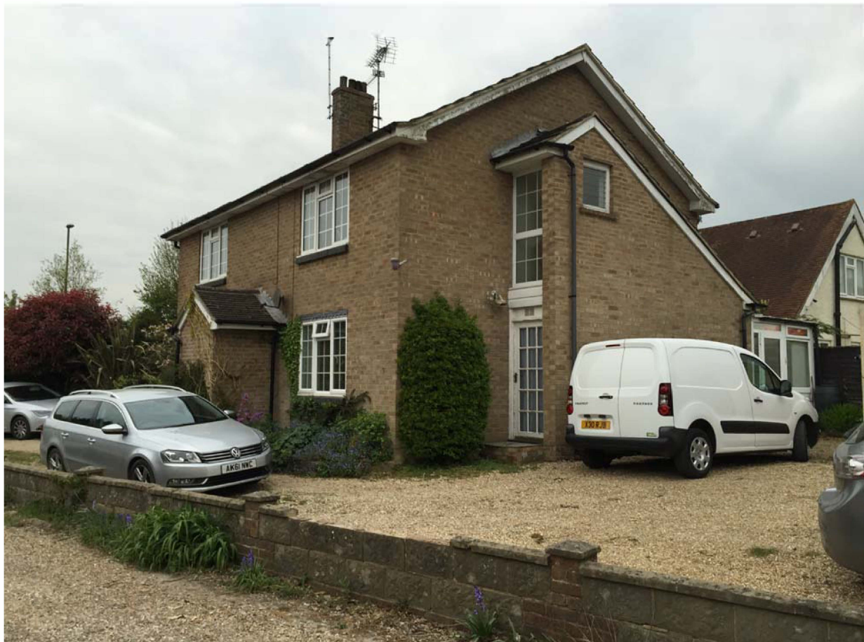
View from the North East - existing access to first floor dwelling
