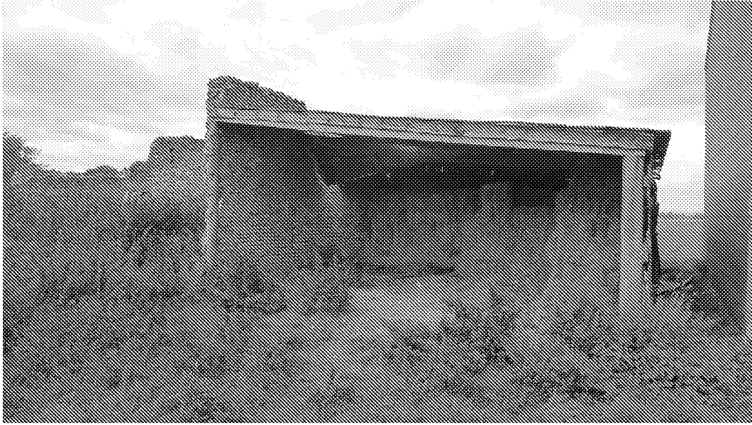
West Shed. Building 3
