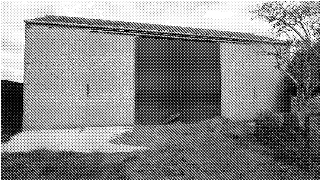
Northwest Barn. Building 2
