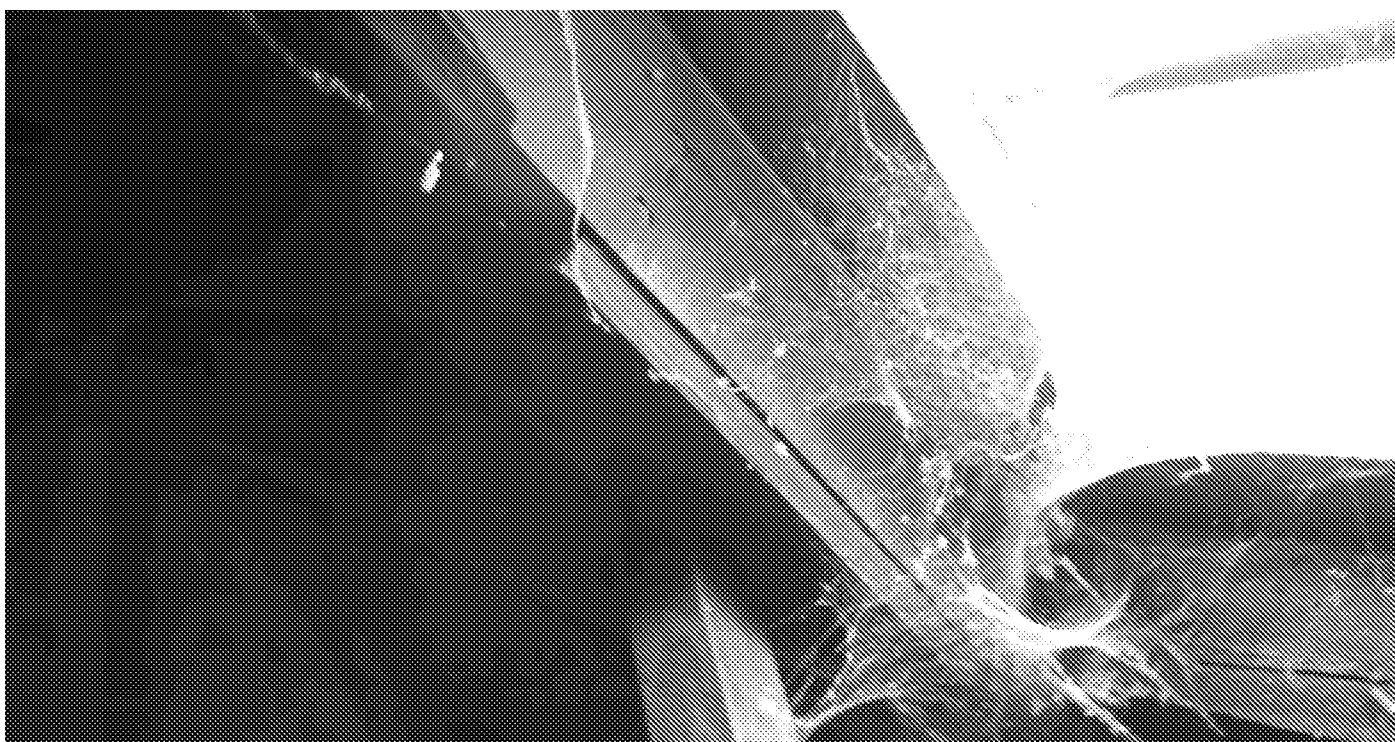
Photograph No. 20 - Heavy cobwebbing and skylight within the loft void of Building B1.
