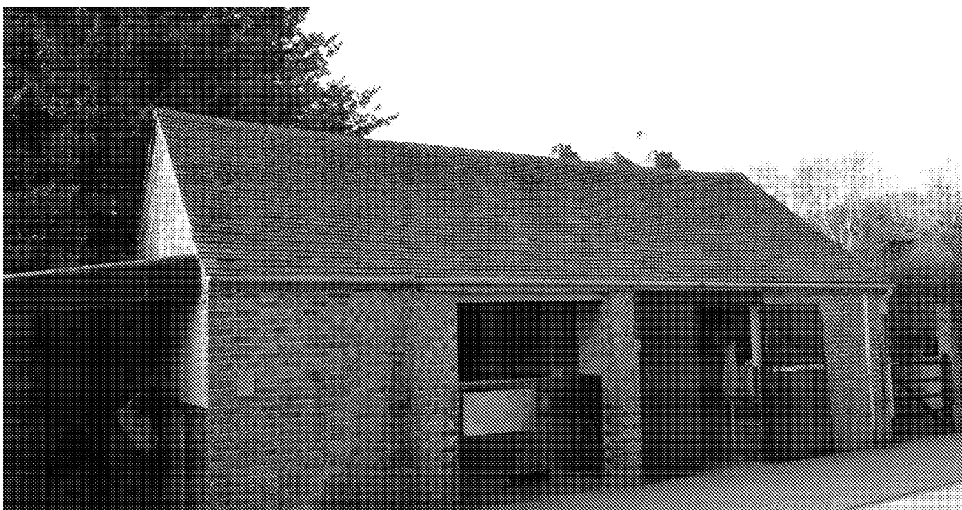
Photograph No. 24 - The traditional stable Building B6.
