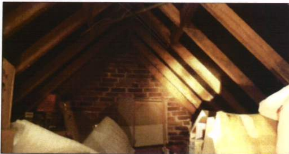
Photo 9: The roof spaces (two roof voids) were carefully inspected for bat droppings
