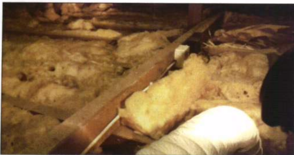
Photo 10: The roof spaces (two roof voids) were carefully inspected for bat droppings
