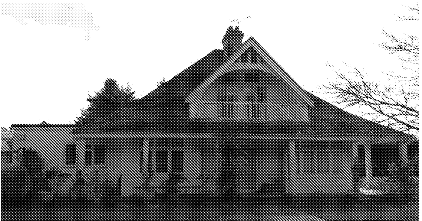
Photograph No. 18 - The dwelling on the site - Building B1.
