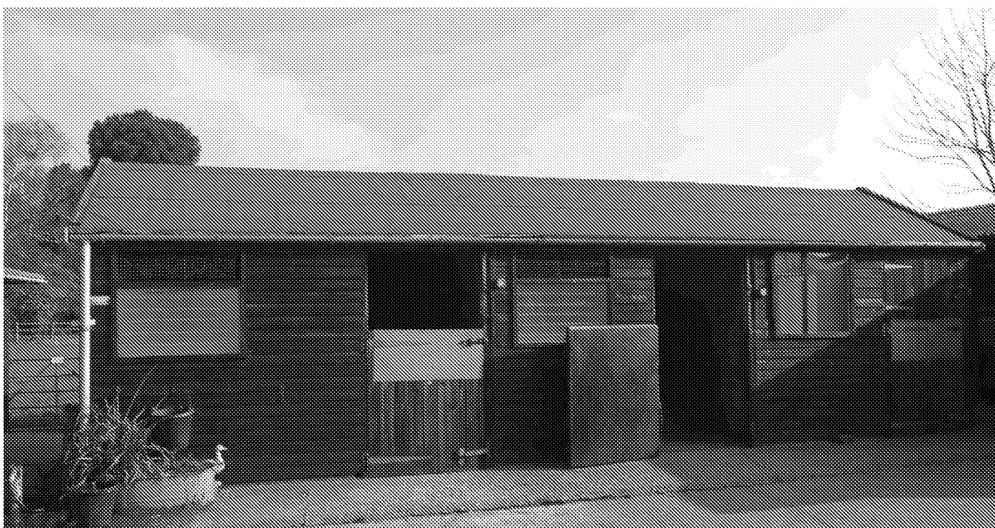
Photograph No. 26 - The stable Building B8.
