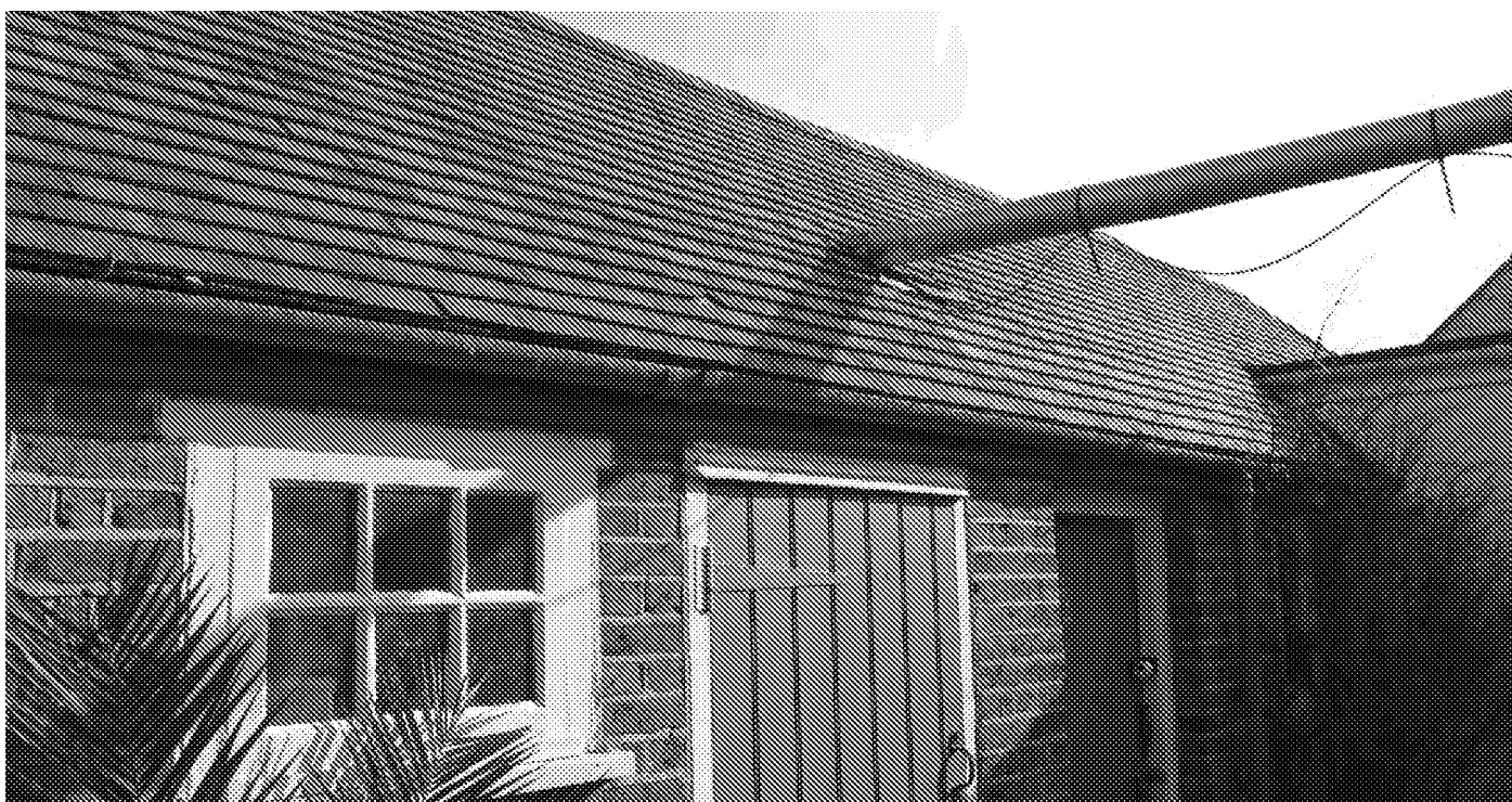
Photograph No. 22 - Buildings B3 and B4 - the store and boiler rooms.
