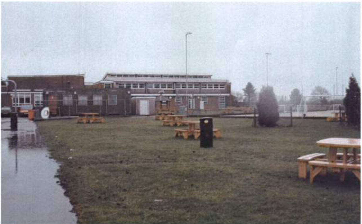
Photograph No. 2 - Existing St Philip Howard Catholic School Buildings.
