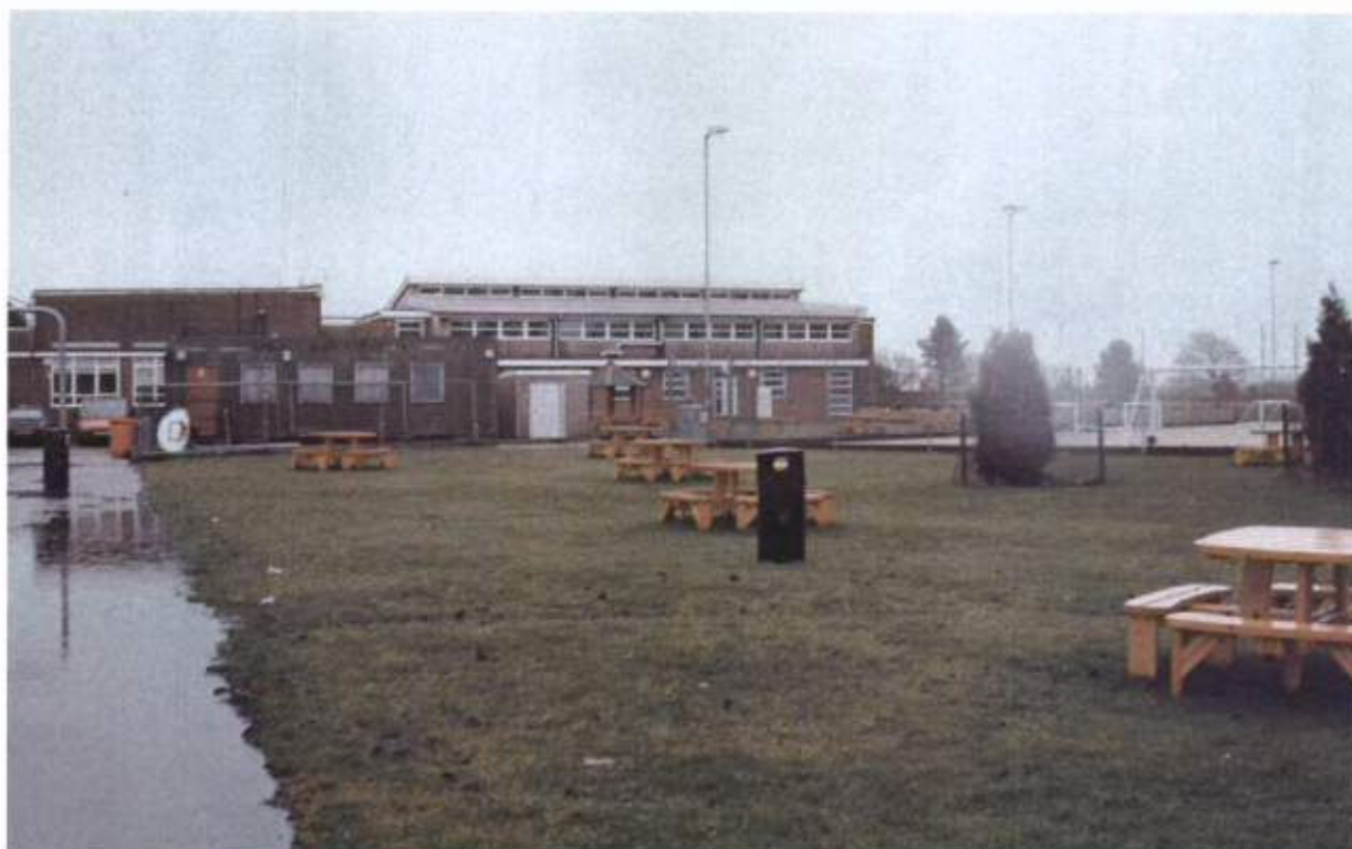
Photograph No. 2 - Existing St Philip Howard Catholic School Buildings.
