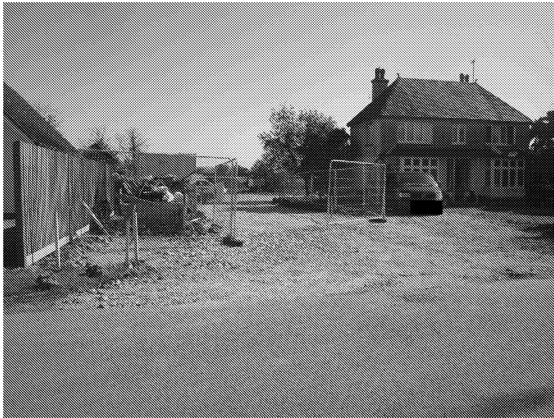
Fig.1 – View NE across site entrance
