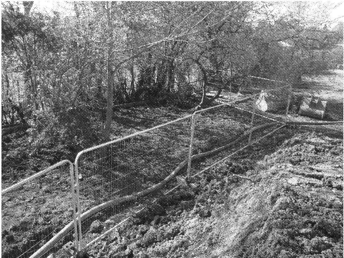
Fig.4 - TPF typical site standard. NE corner of site.
