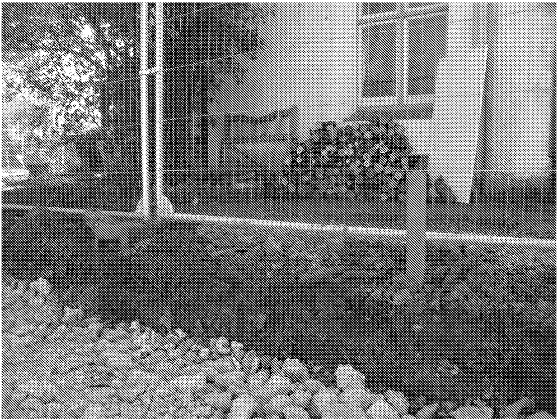
Fig.5 – Excavation continues alongside T25.
