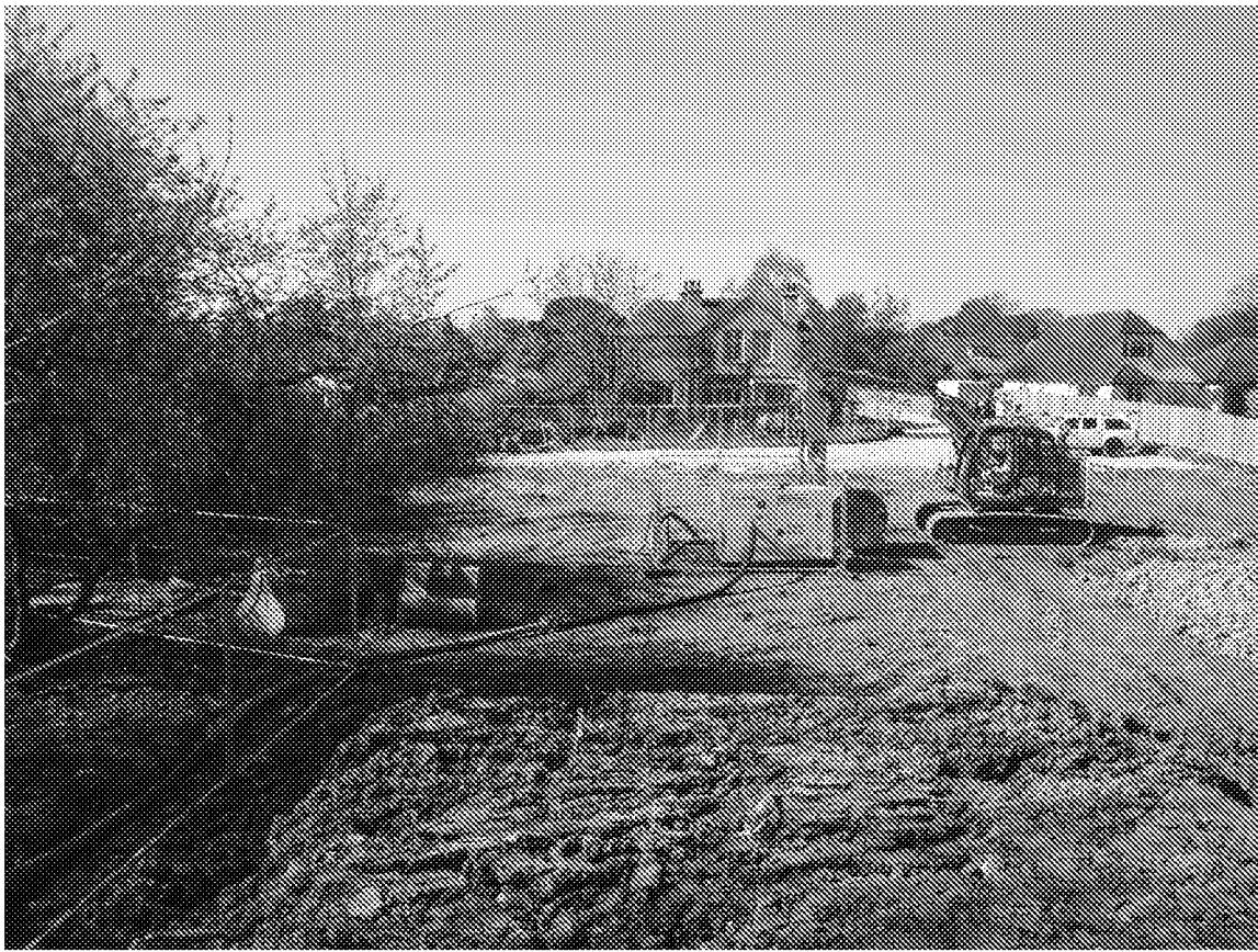
Fig.6 – Looking back towards dwelling from top of soil bund at East end of site.
