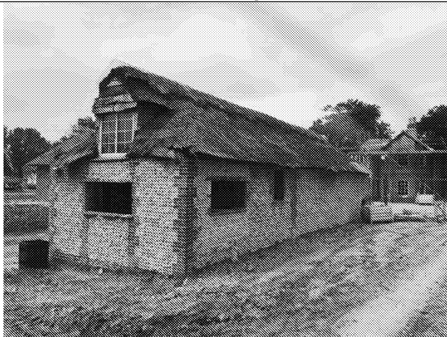
Building B3 The Thatched Cottage viewed from the south-east
