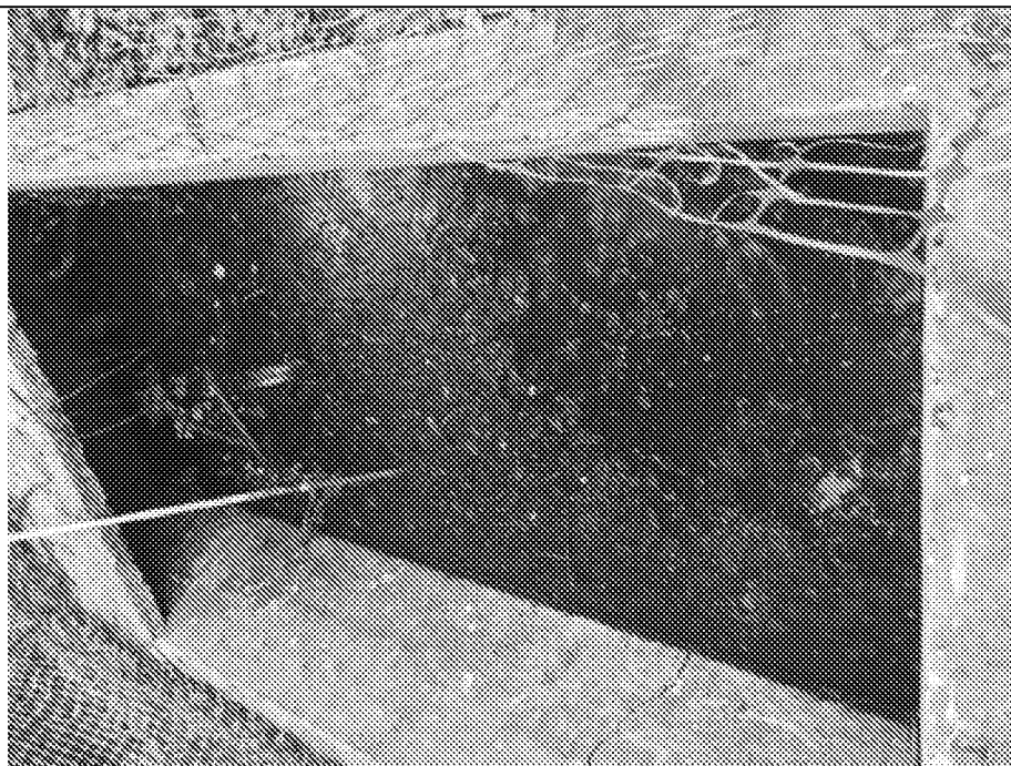
Septic tank to the east of the modern trailer home.
