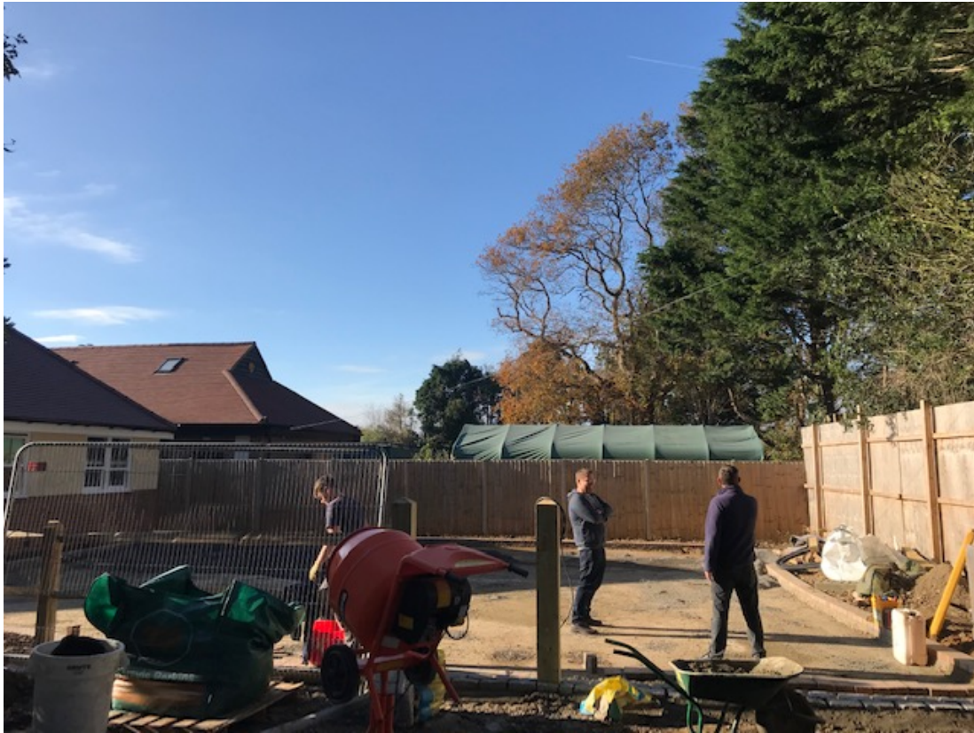
5. Driveway of Winterberry, looking West. House seen on the left.
