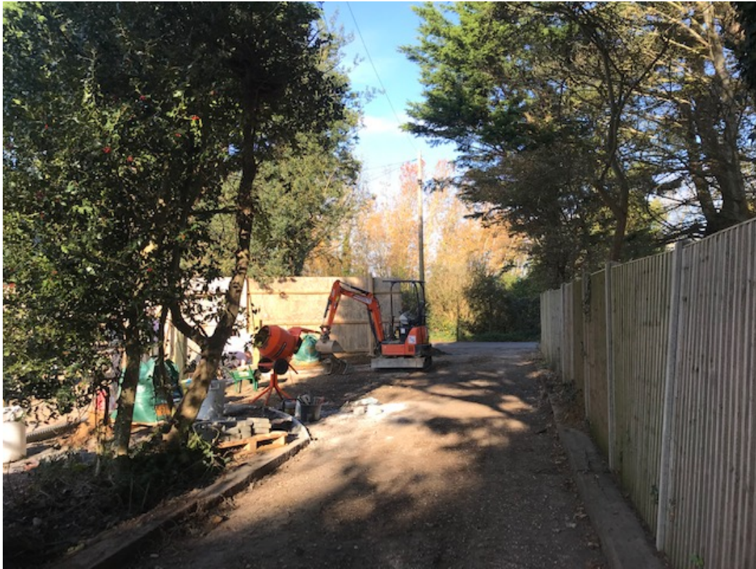
11. View out of access lane, to Horsemere Green Lane. Winterberry access viewed on the left.
