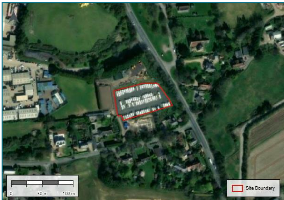
Figure 2.1 – Aerial View of Existing Site
