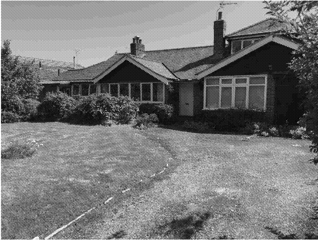
Figure 1 – The front driveway leading from Horsemere Green Lane and the northern aspect of the property Langford.
