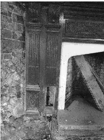
Photographs 6.07 & 6.08 Showing original timber lintel in place but with significant wet rot.
