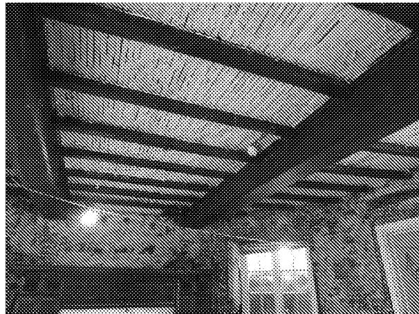
Photographs 6.01 & 6.02 showing the general arrangement with laths remaining insitu and brick piers supporting original timber girders.
