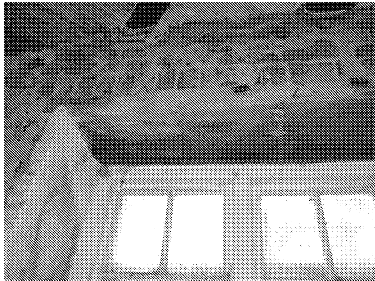
Photographs 6.07 & 6.08 Showing original timber lintel in place but with significant wet rot.
