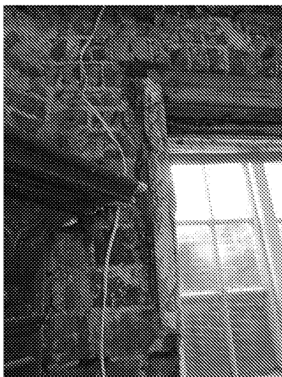
Photographs 6.05 & 6.06 Showing modern timber joists replacing original lintels with little or no bearing onto the original masonry.
