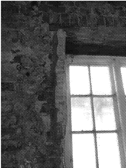
Photographs 6.07 & 6.08 Showing original timber lintel in place but with significant wet rot.
