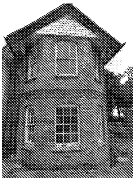
DSC03143 Double Height Canted Bay
