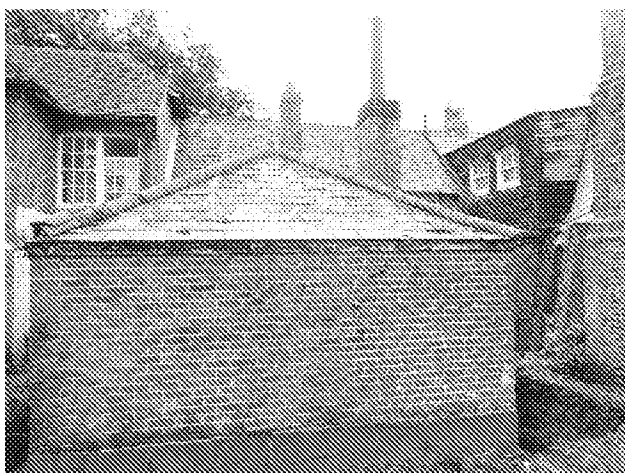
DSC02699 West Elevation
