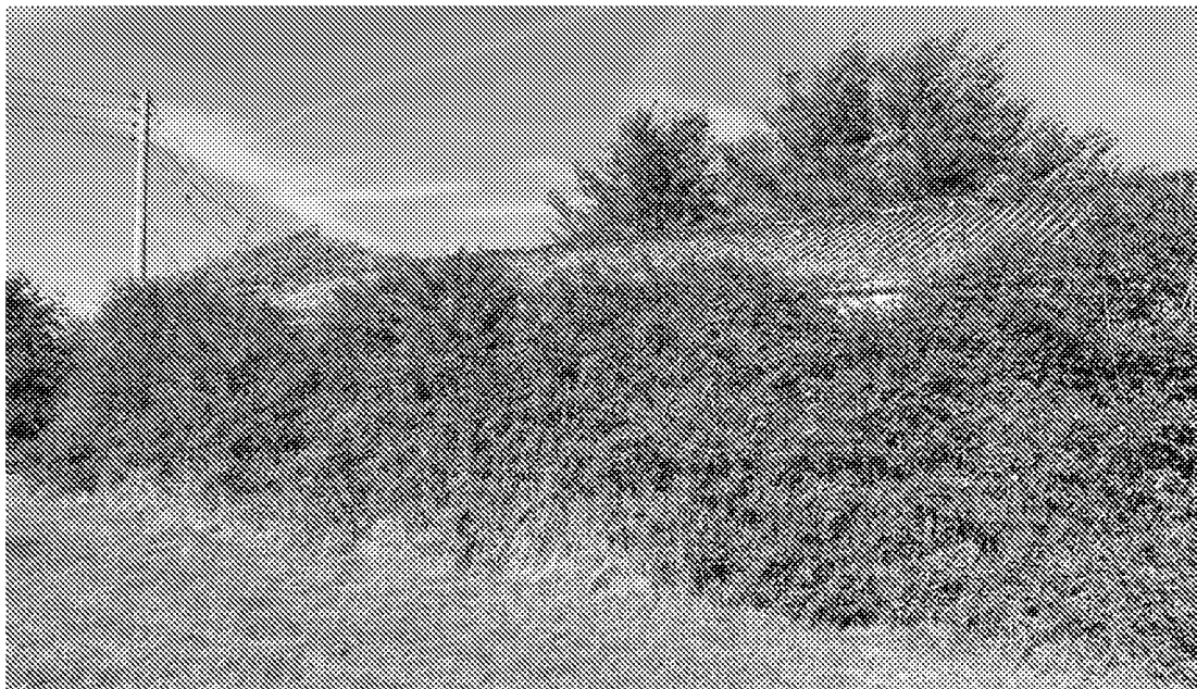
Figure 5.1 Building surrounded by overgrown vegetation
