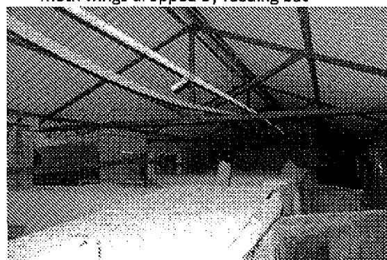
Interior of Building A
