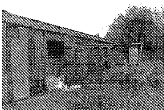
View of Buildings from south west
