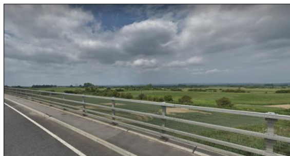
View looking over sub area 1 from the raised carriageway on the A259 ( www.google.co.uk )
