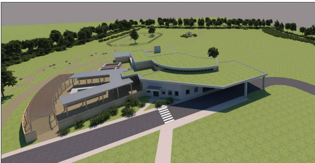
Figure 5: View of the approach to the crematorium building
