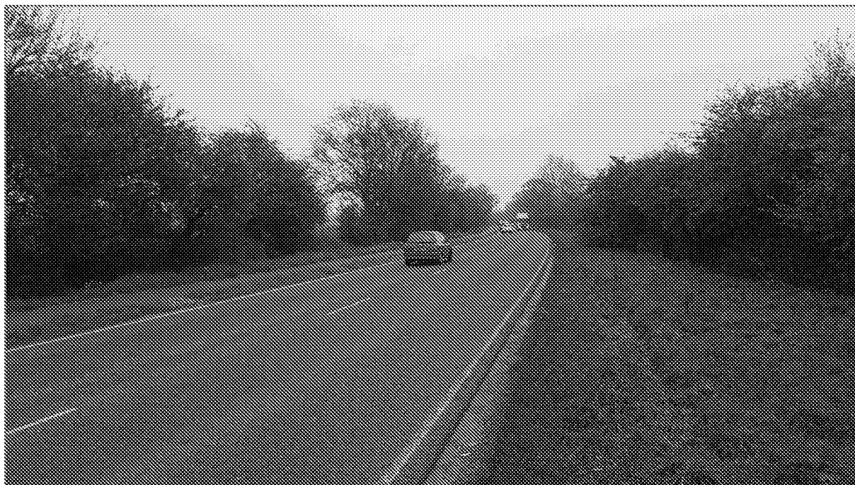
Photo 6 - A259 view east.
