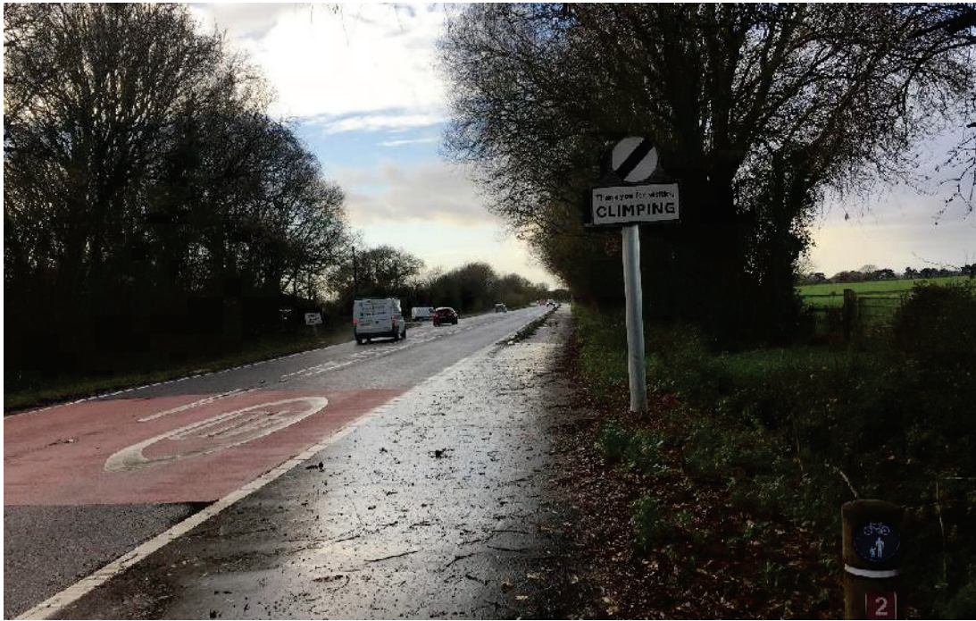
Figure 3-3 Shared cycle / footway along the A259 north of the site
