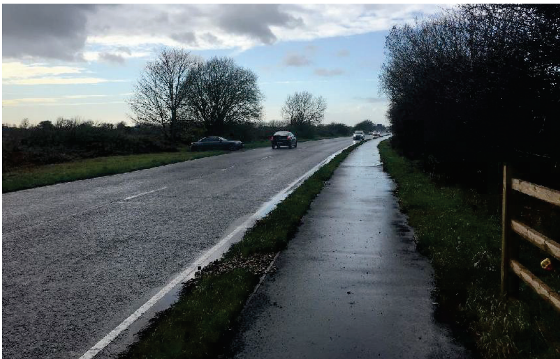
Figure 3-5 Conditions on A259 in the local site vicinity
