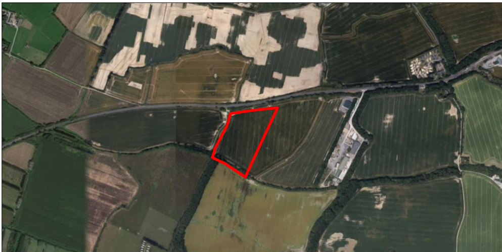
Aerial view of the site ( www.google.co.uk )
