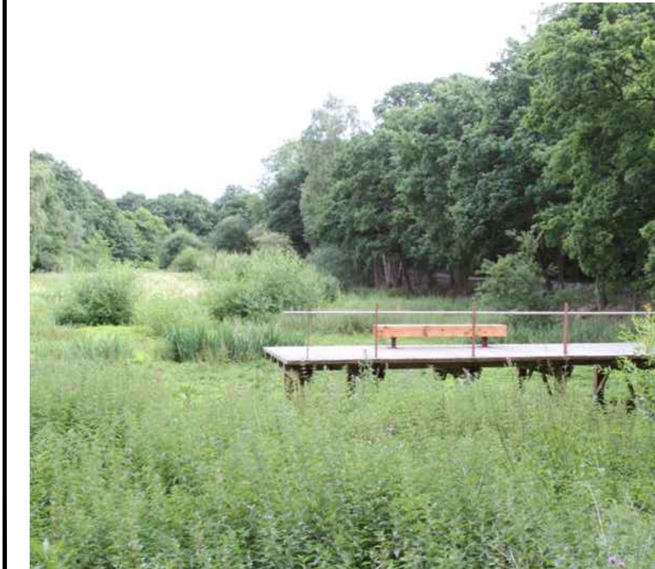
Viewing deck with associated seating, signage, safety line and retaining elements to enable close relationship to water habitats
